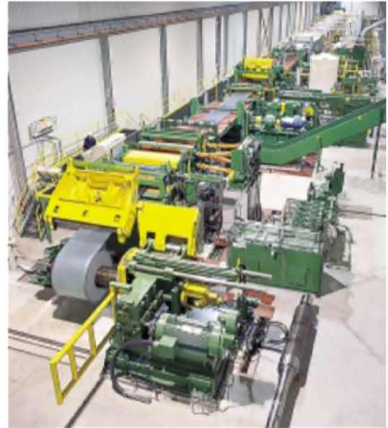
One of Nelson Steel's most recent pickling lines, operating in Canada with a capacity of 450,000 T/A, has some of the most modern features in steel pickling technology.
